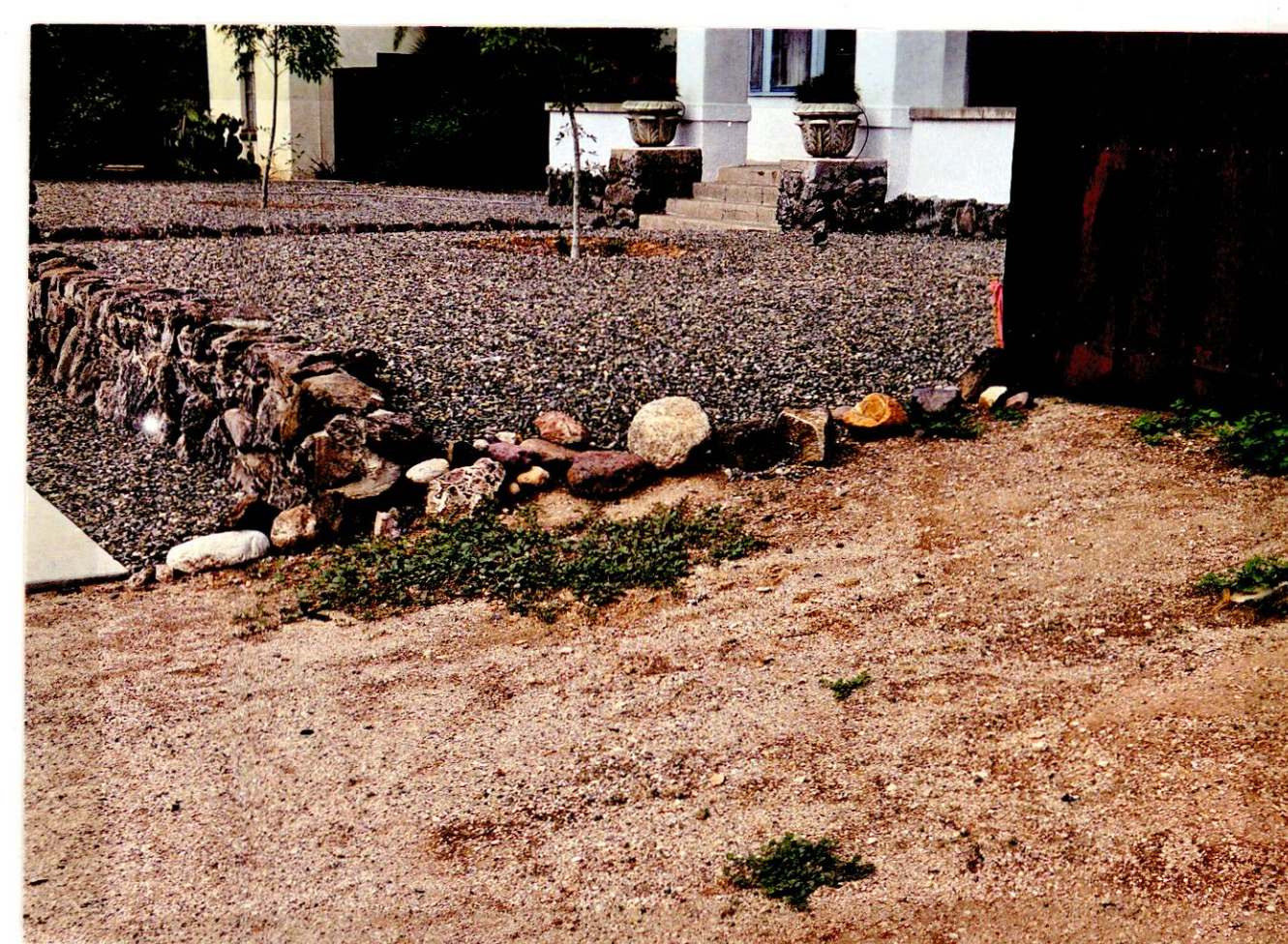
VIEW OF EXISTING EDGE OF PROPOSED DRIVEWAY/ TO BE MORTARED LAVA STONE EDGE.
