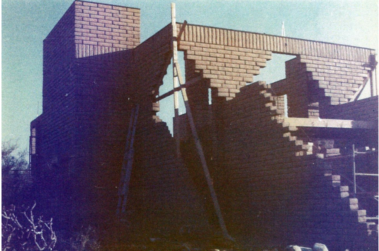
Fig 17. Celestine Barby II House, Under Construction, Current Owner Johnson Collection
