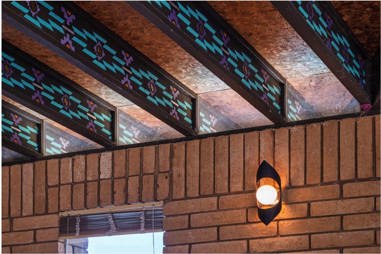
Fig. 11 Celestine Barby II House, Roof Structure, Clerestory, and Stenciled Beams, Photo by GM Vargas 2025
