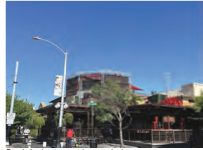
Steel shade structure/ upper deck
