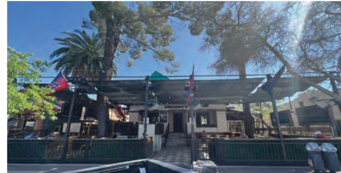
870 E UNIVERSITY BLVD SHADE STRUCTURE
