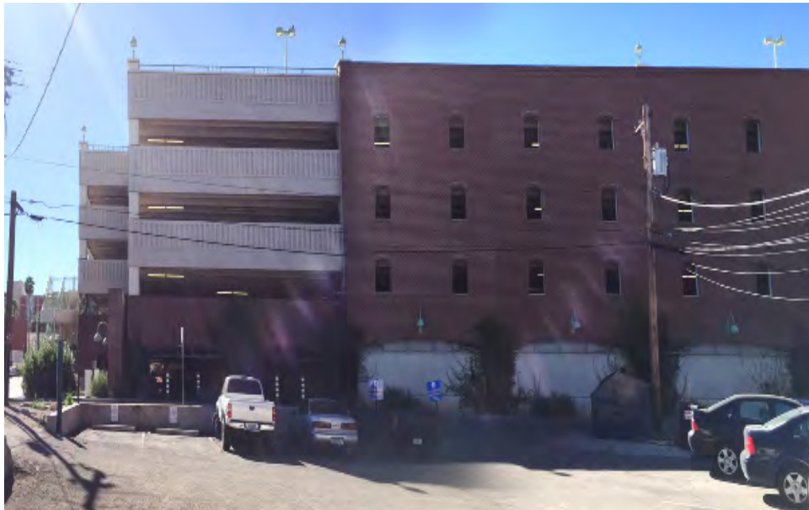
VIEW TO THE SOUTH
