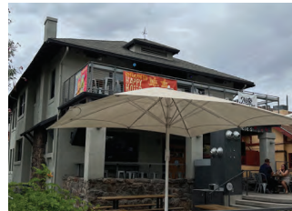
Current view from the corner of University Blvd & Tyndall Ave
