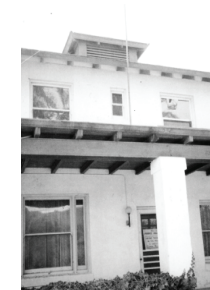
NORTH ELEVATION DETAIL
