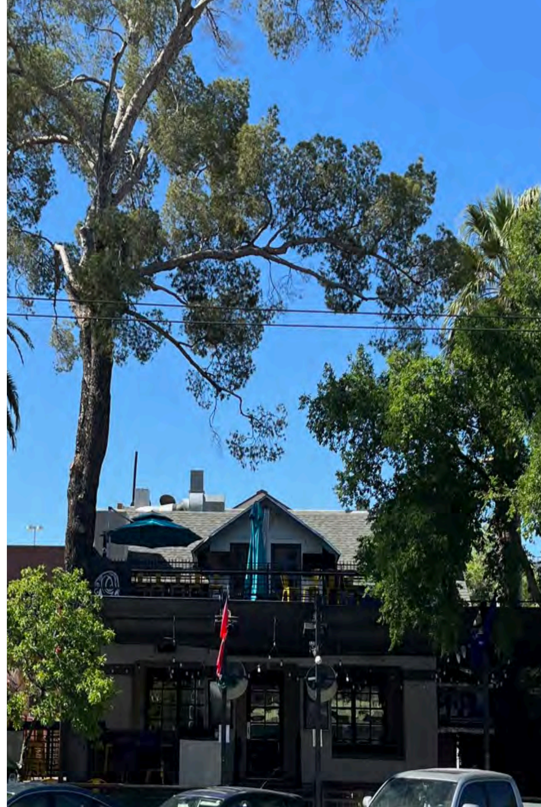
870 E UNIVERSITY BLVD UPPER DECK WITH SHADE
