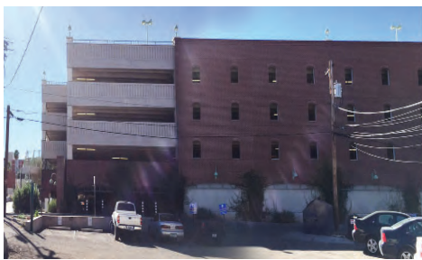
VIEW TO THE SOUTH
