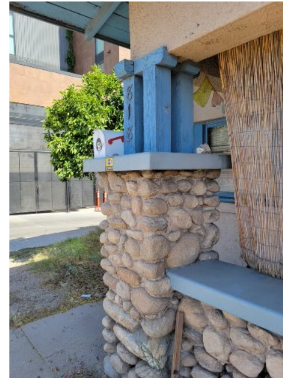
Porch pier, east end. Identical spacing to west pier.
