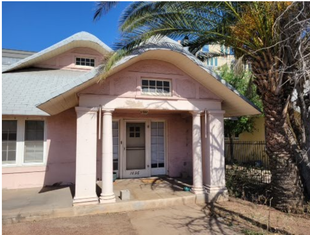
Porch piers and columns, west facade, with jerkinhead gable.
