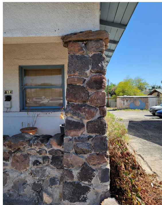
Detail of tufa stone pier and soffit
