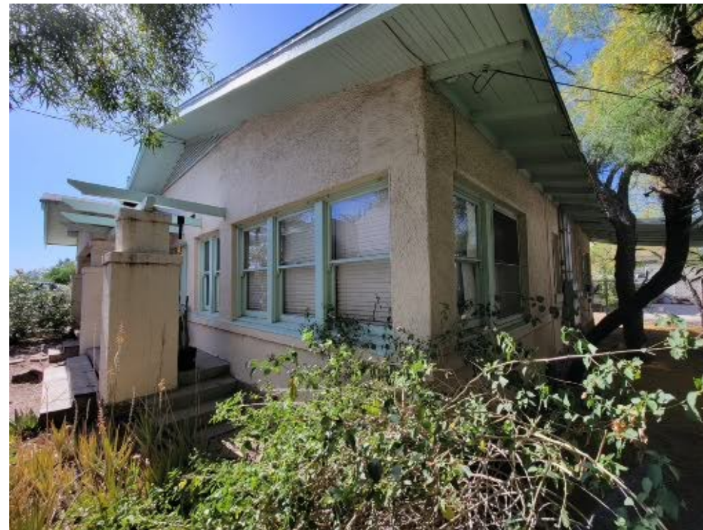
South elevation, looking west from SE corner. Pergola is dominant feature.
