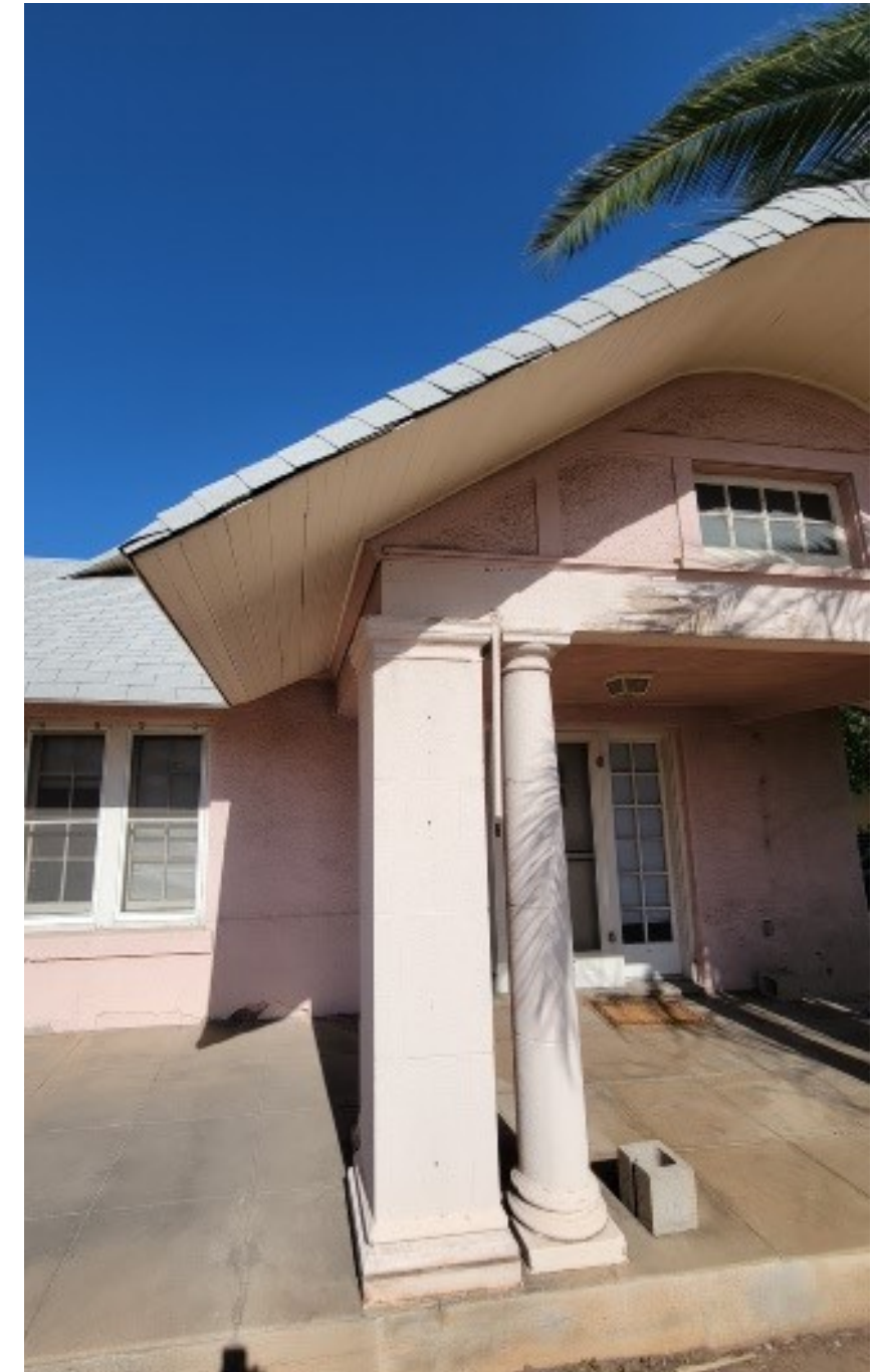
Porch pier is stucco with a scored ashlar pattern etched on surface.
