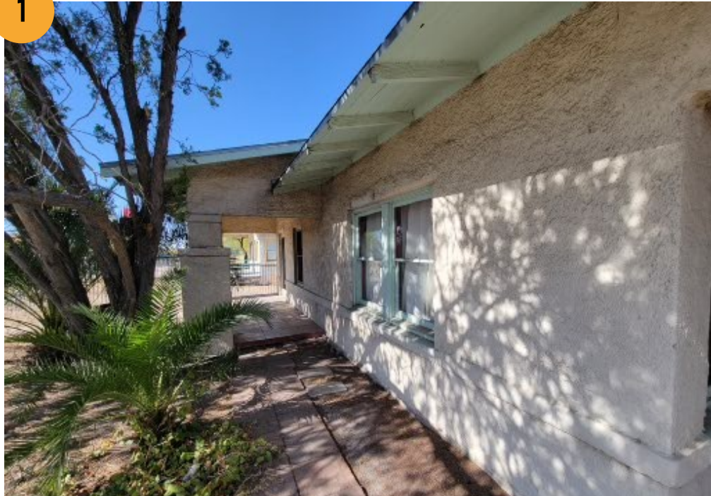
Front - West Elevation (view looking north)
