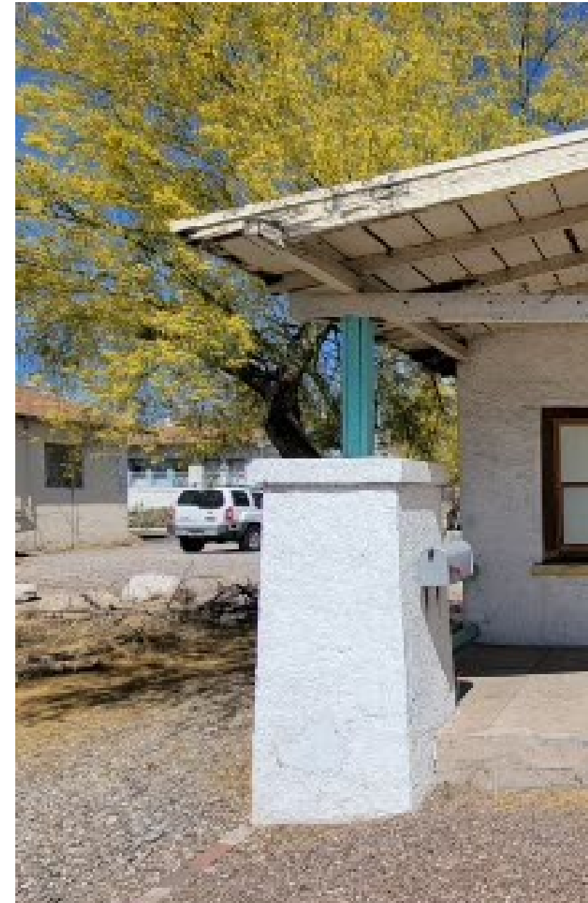
Porch pier, north side. Note very minor taper in form. 77" high.
