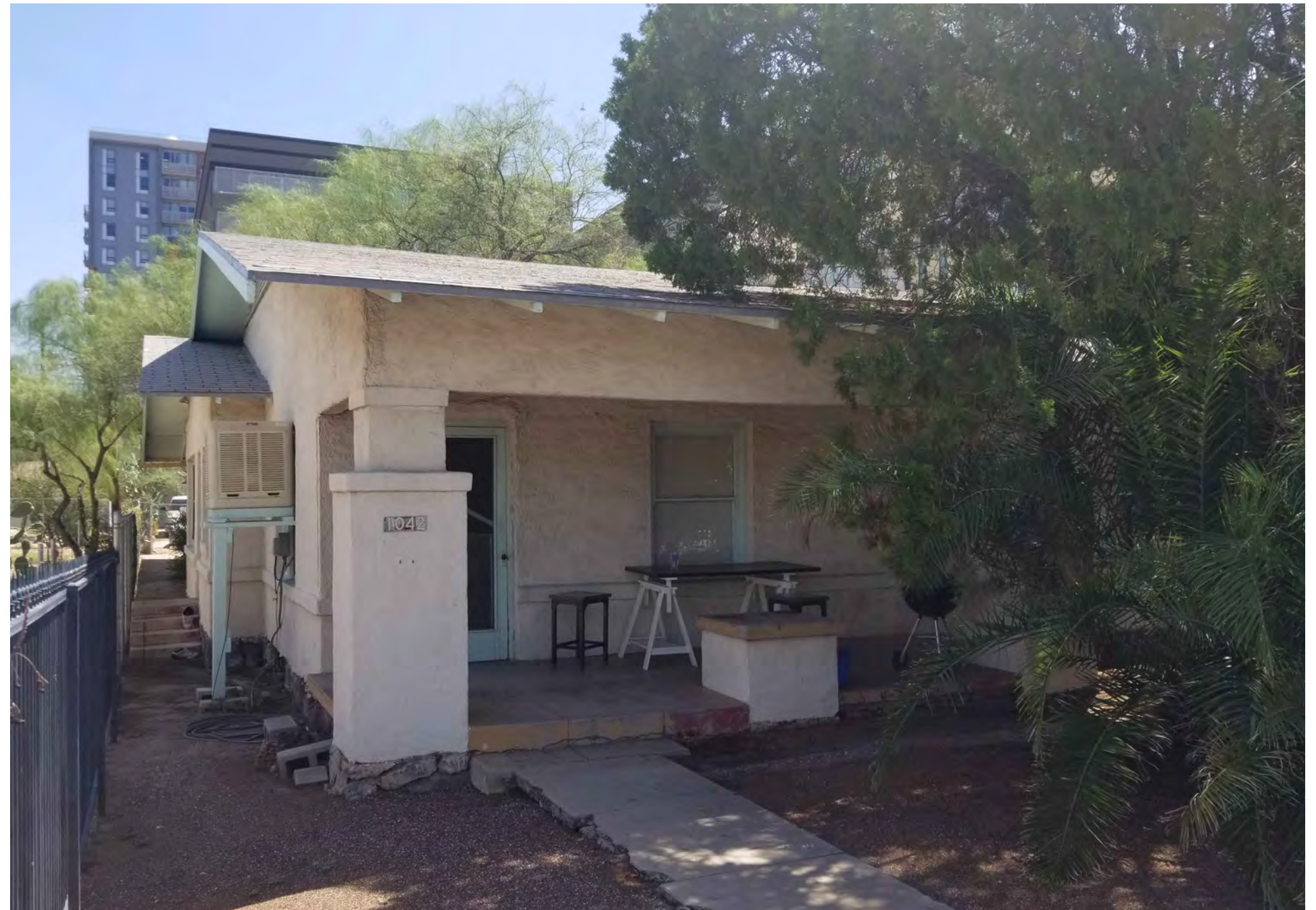
North Entry (1042) and Porch facing Euclid.
