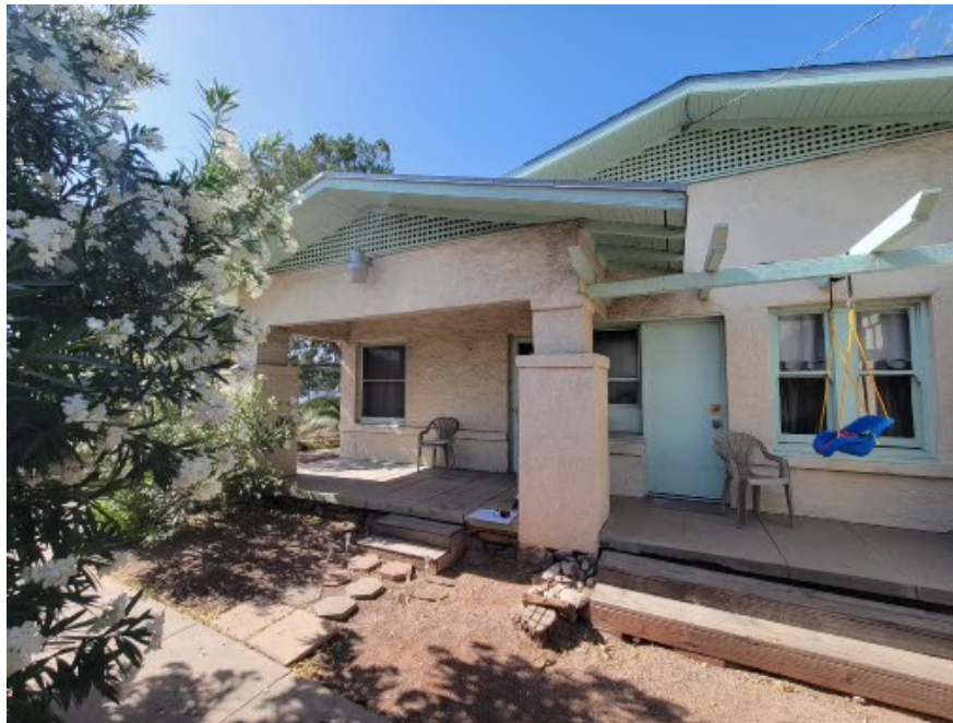
South elevation featuring porch
