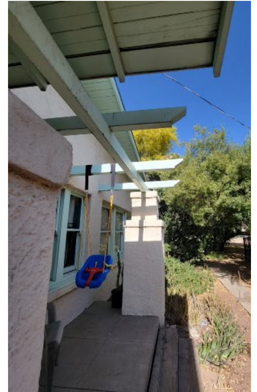
Detail of pergola on south elevation. View to east.
