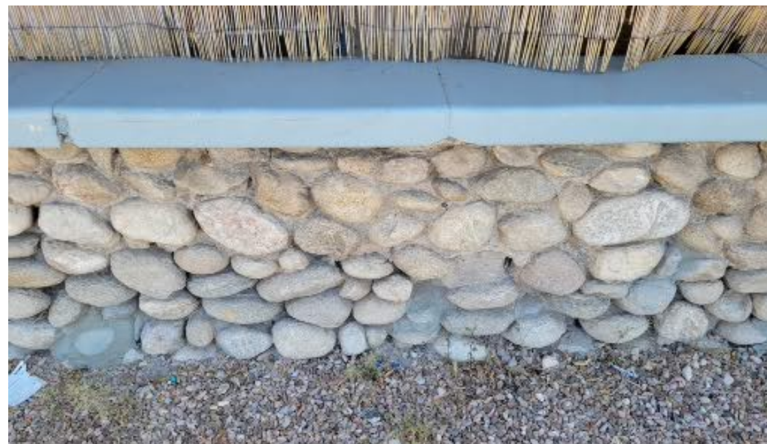
Cobblestone spacing, front face of porch wall.
