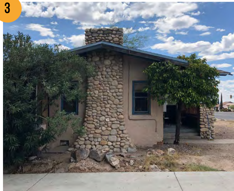
East Elevation featuring cobblestone chimney
