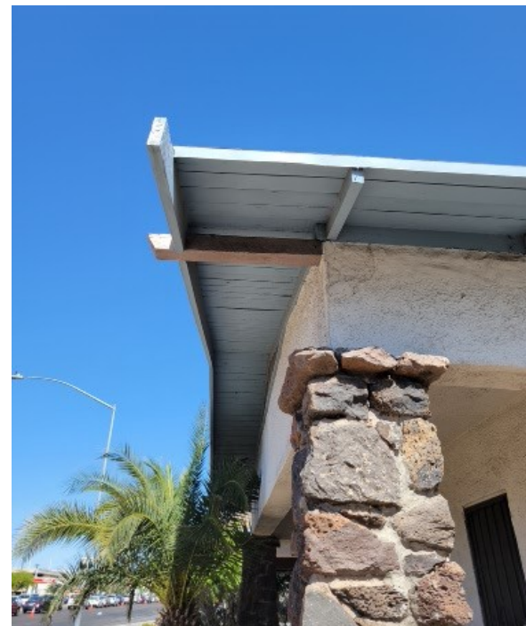
West porch pier and 1'6" soffit
