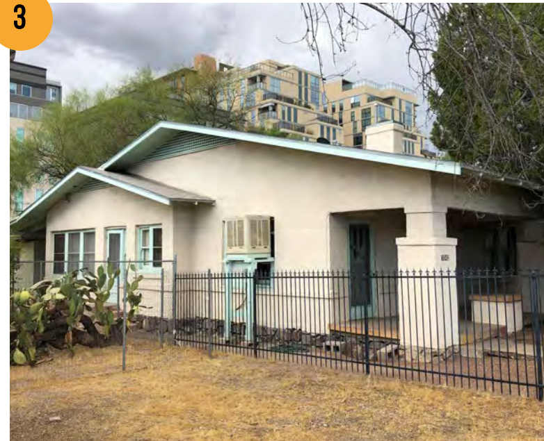
North Elevation (looking southeast)
