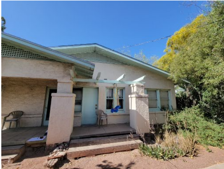
South elevation with porch and pergola
