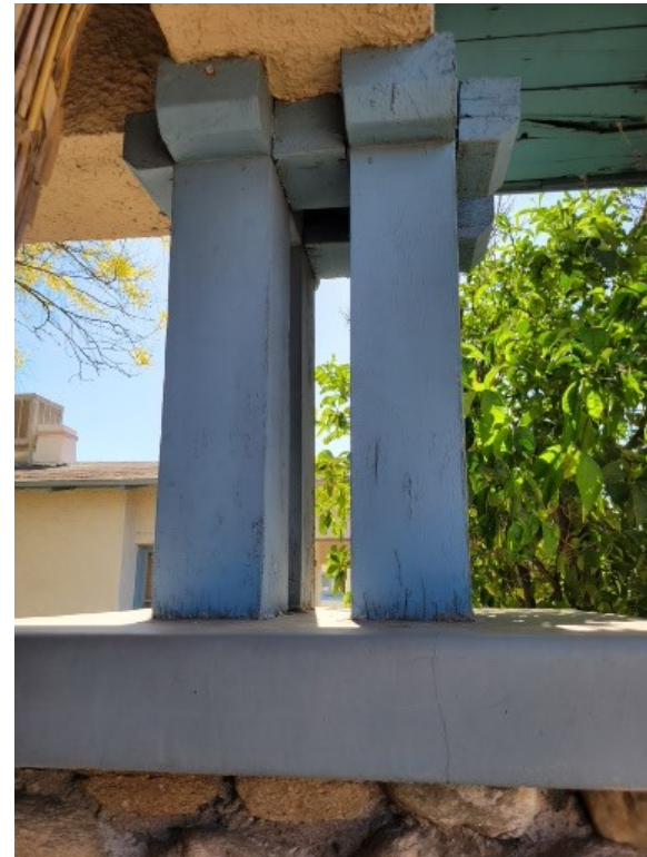
Detail of posts, looking west on west pier
