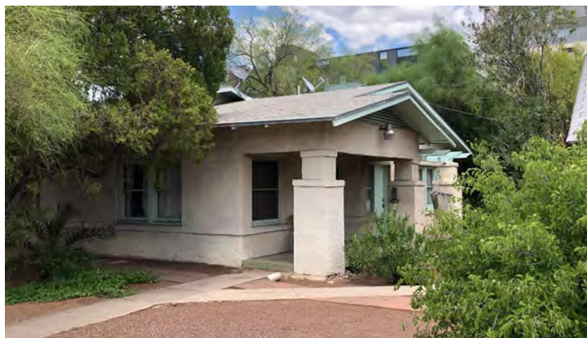
South Entry (1040), facing south, side yard.
