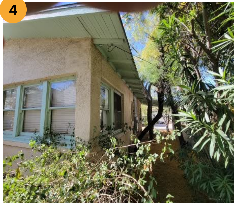
Southeast Corner, east (rear) elevation.
