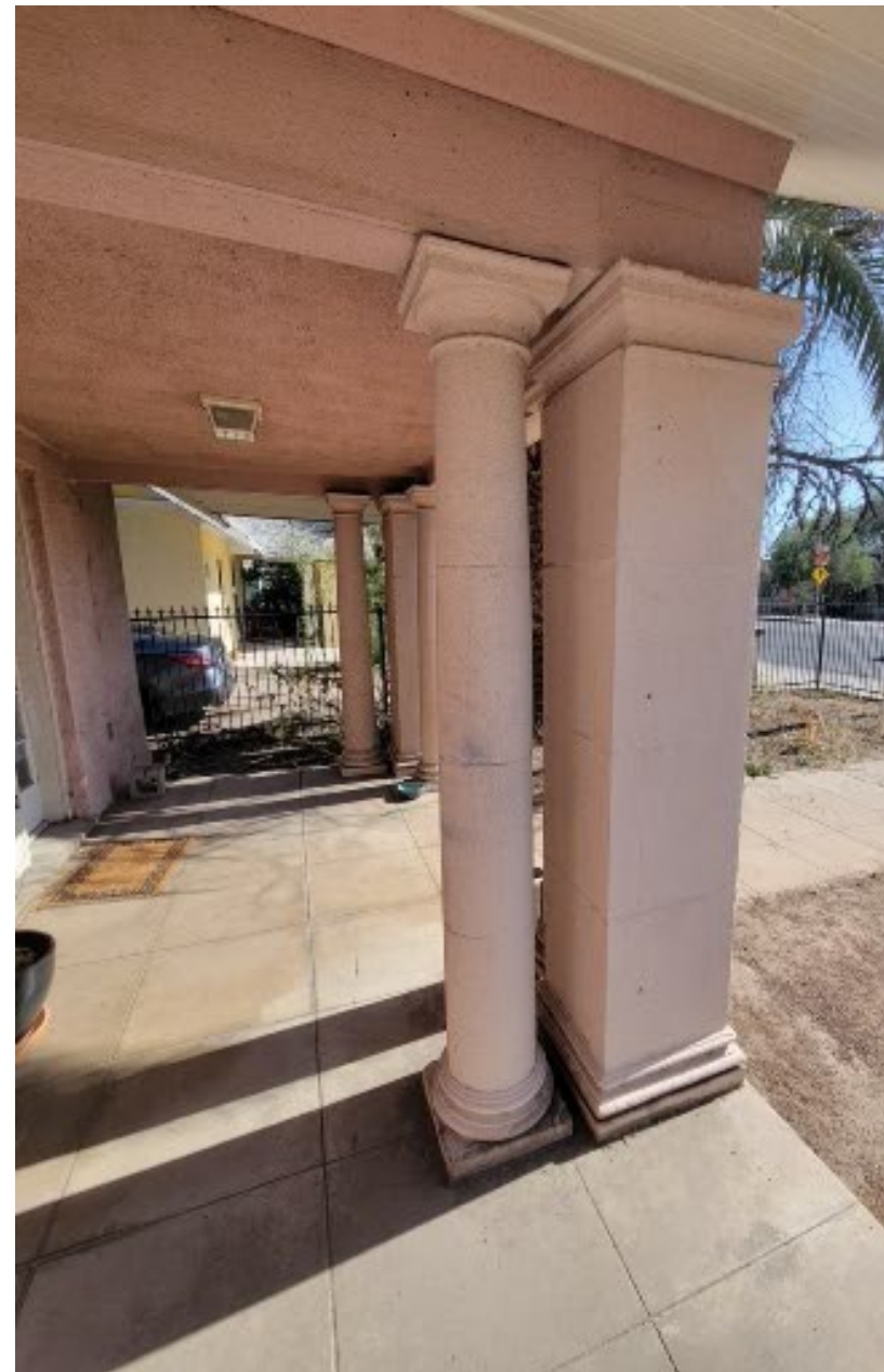
Porch piers and columns. Note slight taper of column, Astragal moldings at base and at Doric capital.
