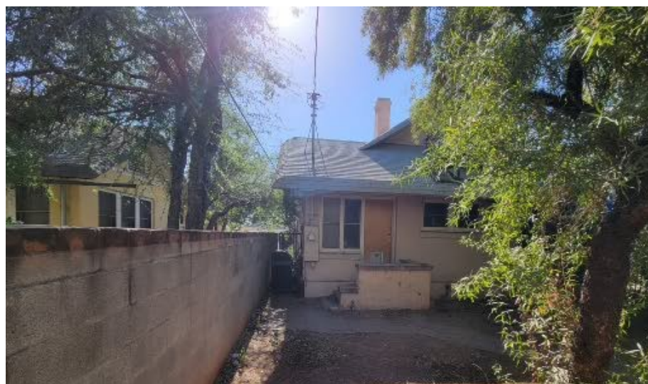
Southeast corner and portion of east (rear) elevation.
