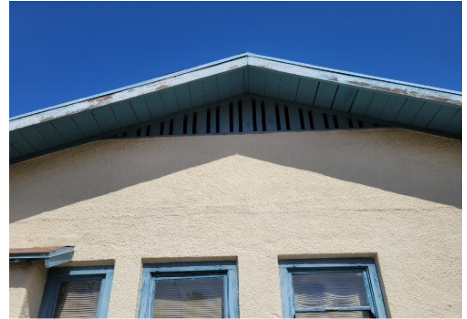
Wood gable vent in west elevation, east gable vent is identical
