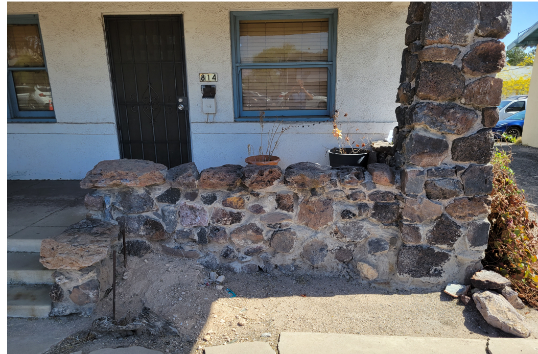
Detail of porch wall and tufa placement.
