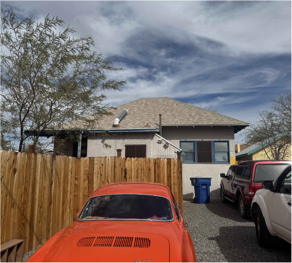
EXISTING WEST ELEVATION W/ SITE FENCE
