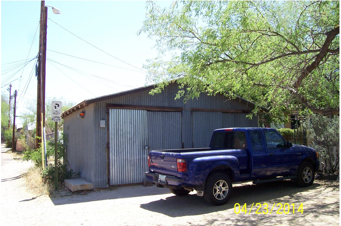
(E) GARAGE THAT HAS BEEN DEMO
