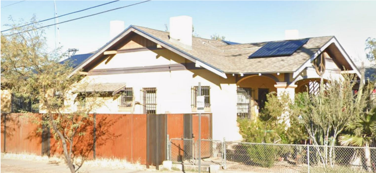
CORRUGATED METAL FENCING, 603 N 3rd Ave.
