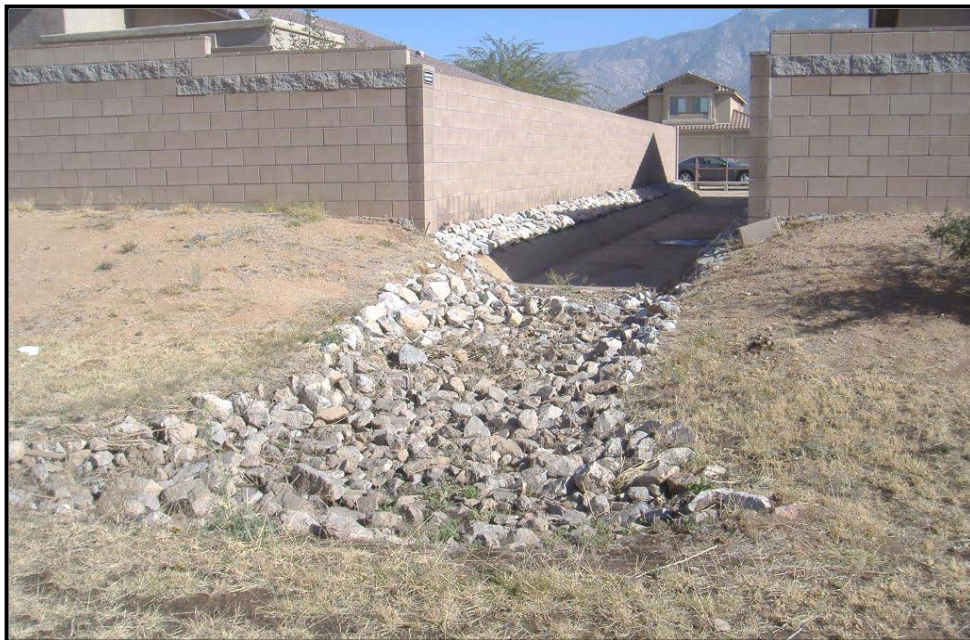
Photo 4.1 Basin Inlet with Riprap Protection
