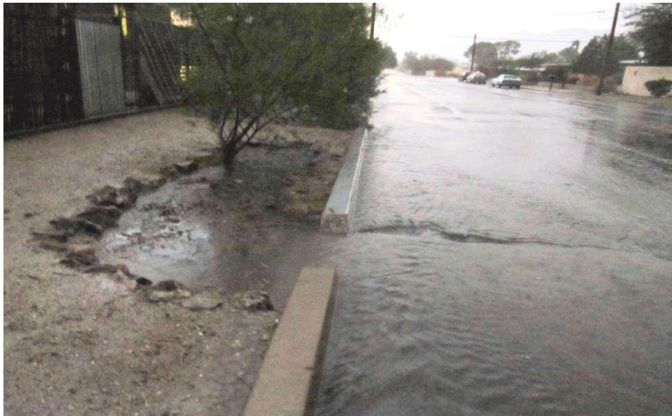
Photo 2.1 Roadside Stormwater Harvesting Basin at Full Depth
