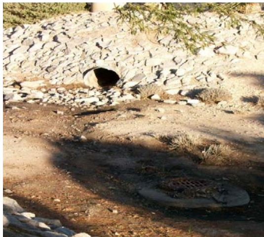
Photo 4.5 Detention Basin Dry Well Installation
