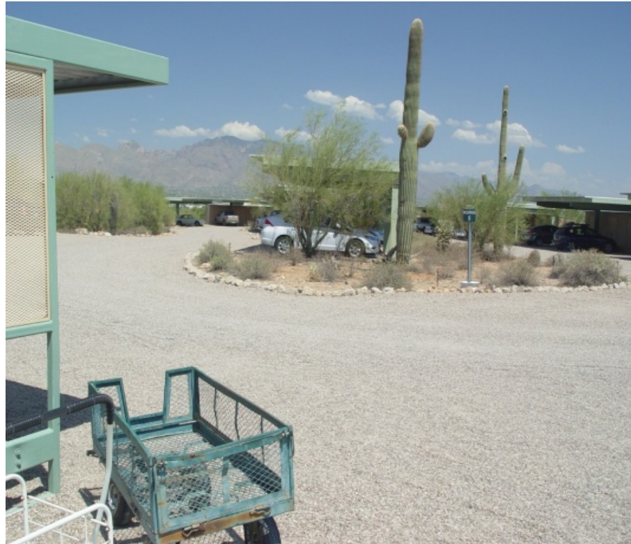
Photo 5.1 Porous Gravel Installation
