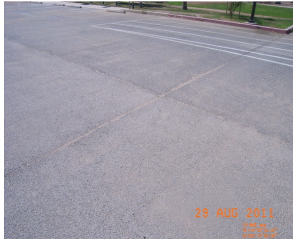
Photo 5.4 Pervious Concrete Installation
