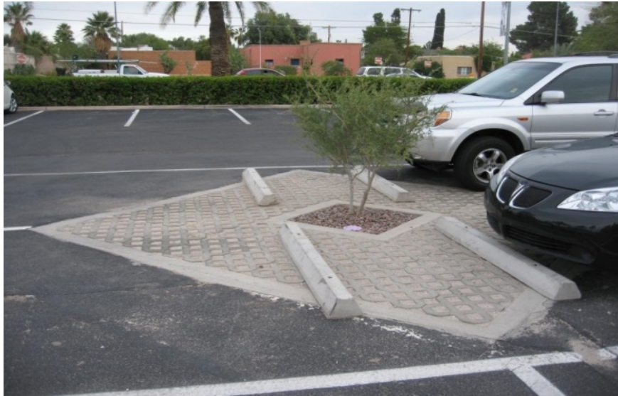
Photo 5.2 Concrete Grid Pavement Installation
