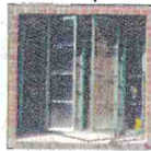
steel casement windows
