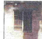
expressed lintel with sloped sill
