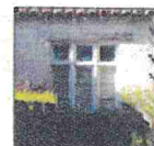
ganged windows with expressed lintel
