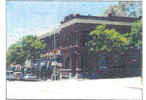
Example along south side
