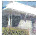
gutter and downspout
