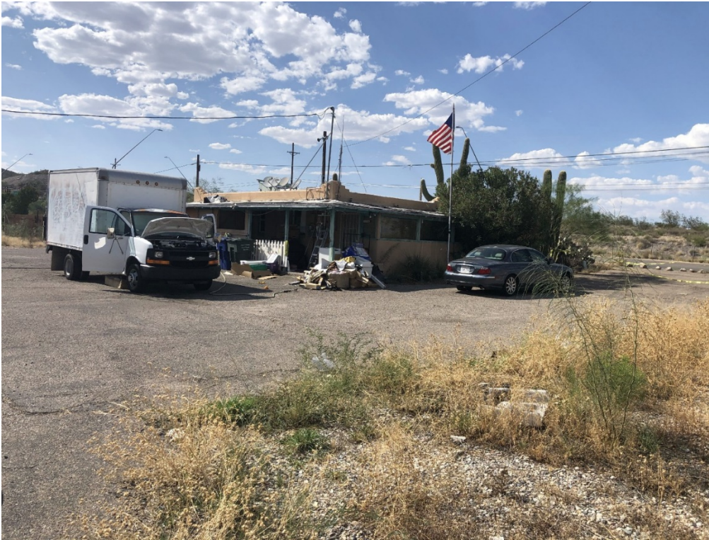
Building A Looking NW
