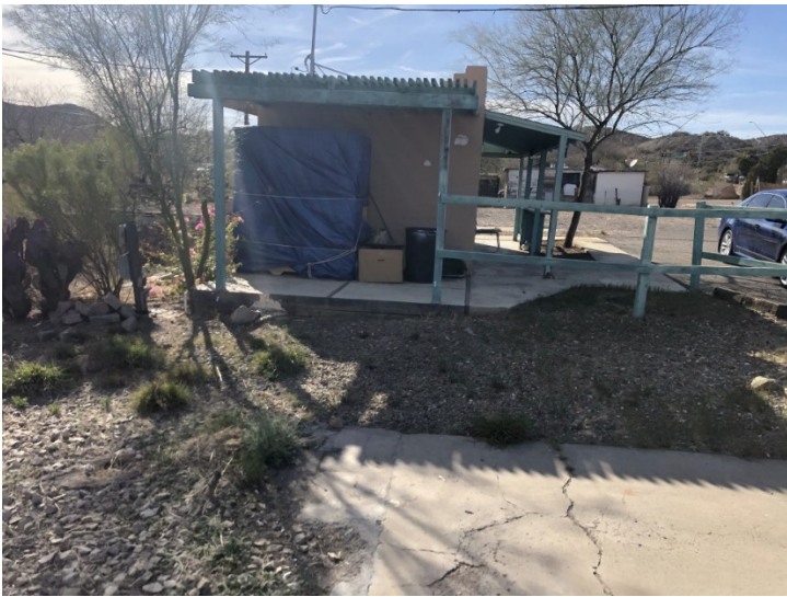
Building B Looking West
