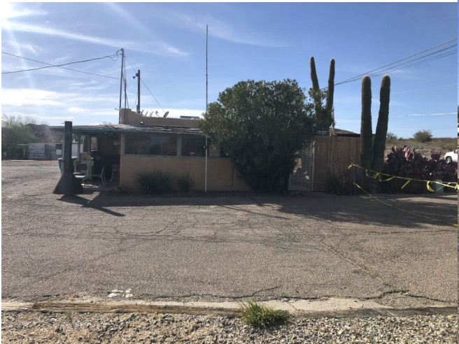
Building A Looking West
