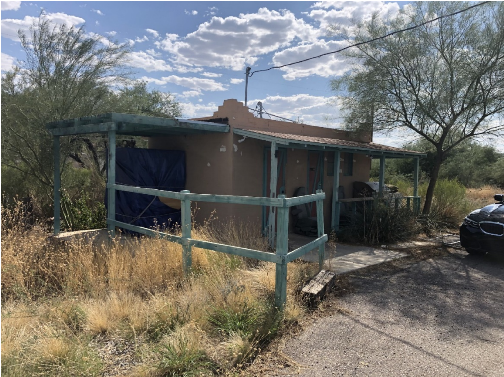
Building B Looking SW
