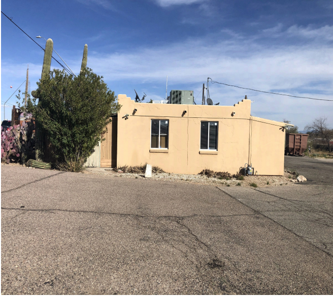
Building A Looking East
