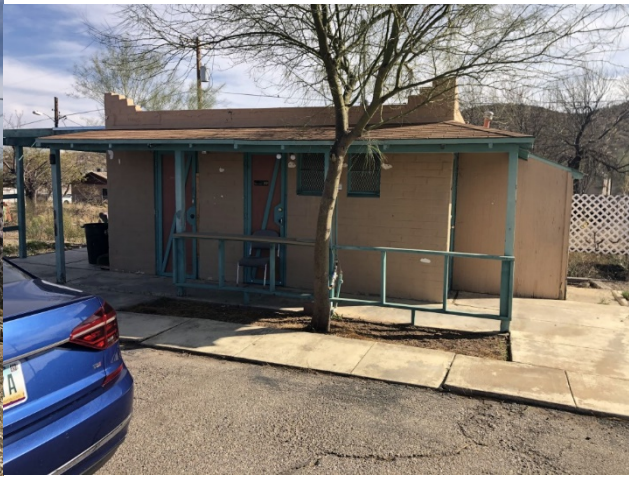
Building B Looking South
