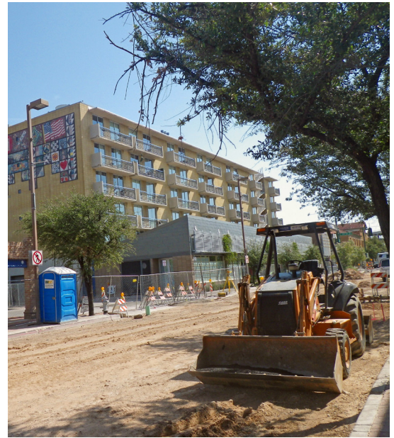
Construction of the Modern Streetcar in Downtown Tucson.
