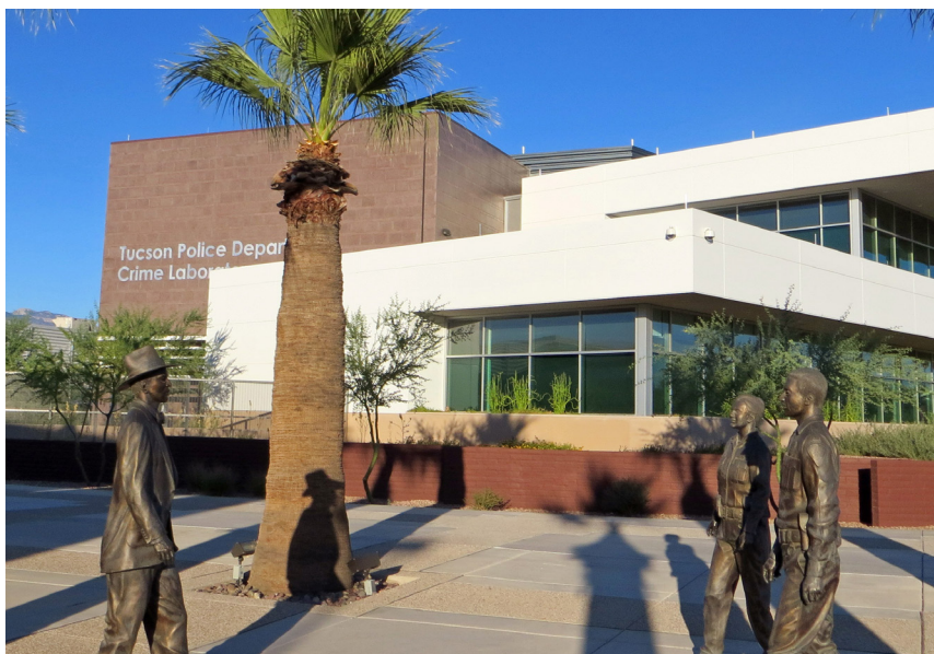
The 62,377 square-foot Tucson Police Crime Laboratory, built in 2011, holds lab and office space for forensic analysts. Energy conservation and water harvesting were key elements of its design.
