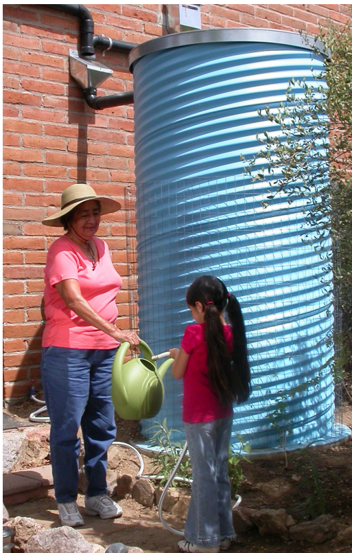
A rain water cistern captures water for non-potable use.
