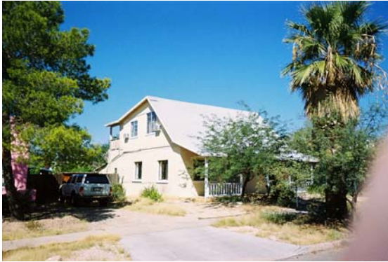
Steeply pitched gable roof
