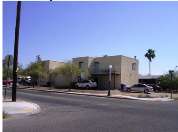
Flat, unrelieved parapet
