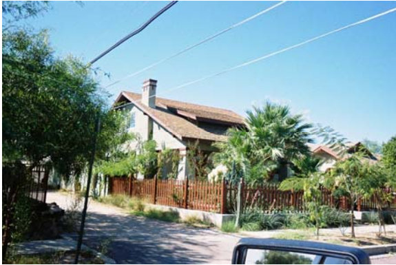
Gable roof with shingles and dormer
