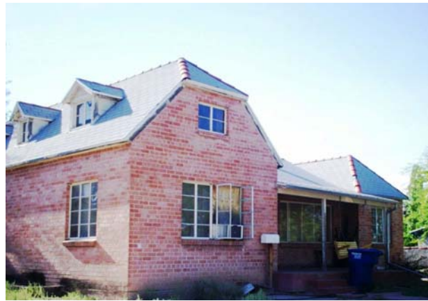
Steel casement windows
