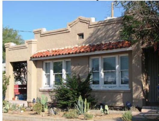
Parapet with detail and varying heights
