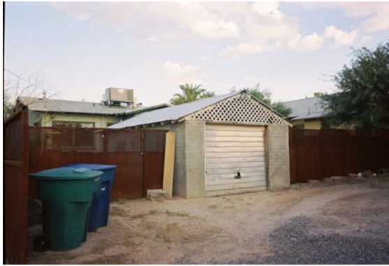
Garage off of alley
