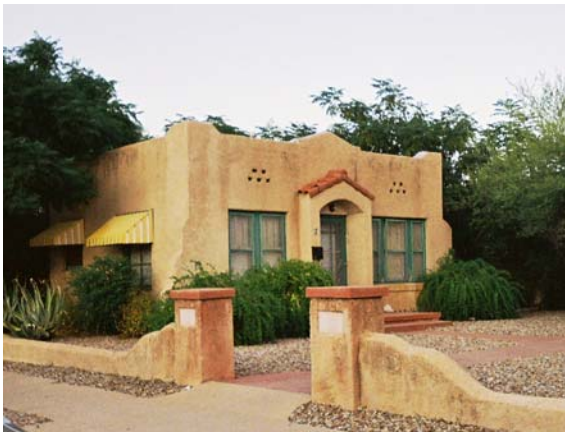
Wood double-hung windows
