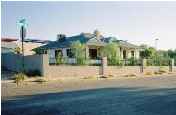
Hip roof with shingles, multiple ridges
