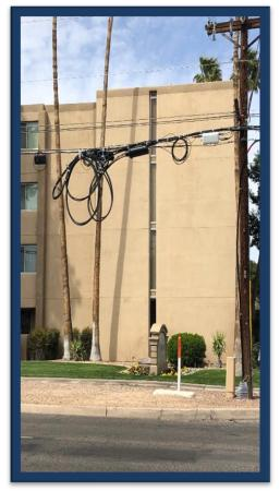
Figure 8 - Excess Overlashing
