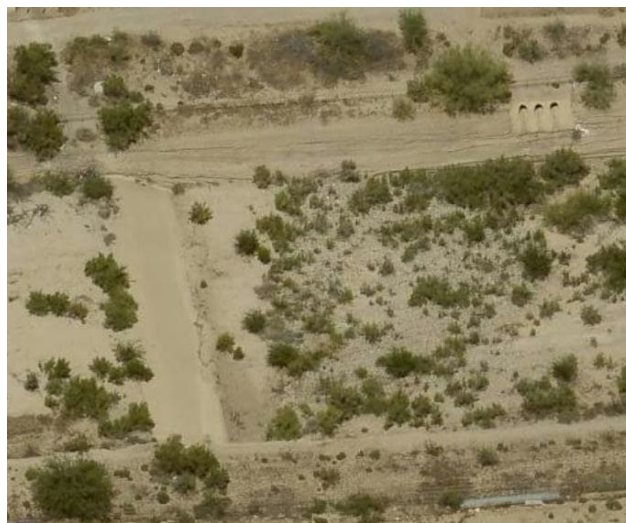
Figure 29: After – Colored concrete protected sewer line
