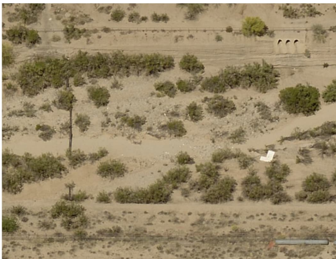
Figure 28: Before - Exposed Sanitary Sewer
