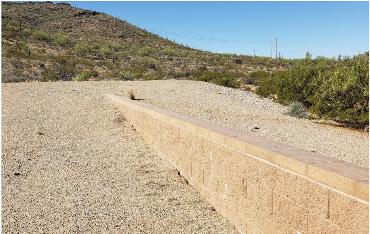
Figure 54: Floodwall Levee on the Silvercroft (ERZ) watercourse at termination point (see page 39)
