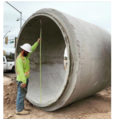
Figure 42: Broadway Boulevard Project includes installation of sixteen 90-inch diameter underground stormdrains as part of the Broadway Improvement Project from Euclid Ave to Country Club Road including approximately 192 tons of stormdrain pipe installed in one day.
