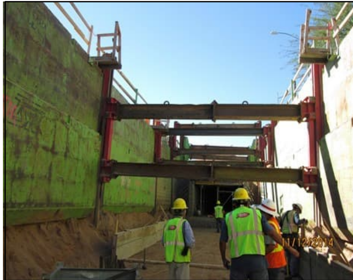
Figure 41: Construction of High School Wash stormdrain
