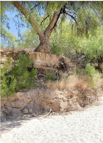
Figure 57: Tanque Verde Creek side slope
