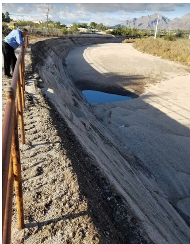
Figure 10: Rillito regional watercourse soil cement embankment with railing and naturally sandy bottom.
