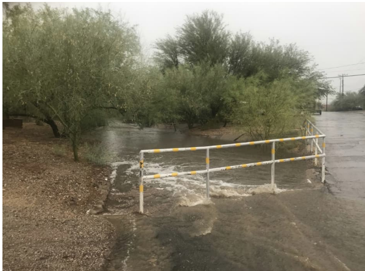
Figure 49: Streets are part of the urban stormdrain system (J. Hayt)
