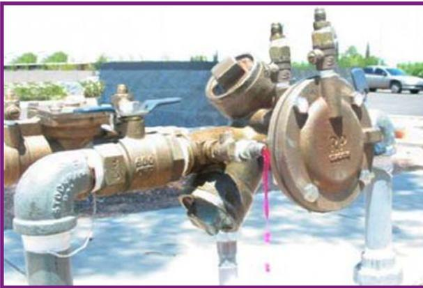
*Figure 6: Colored water at the number 4 test cock indicates a cross-connection*
