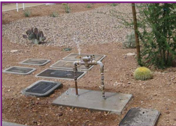
Figure 2: Draining water pressure through test cock #4
