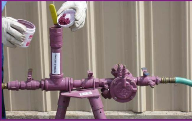
*Figure 3: Dye is added through dye port on the temporary jumper assembly*
