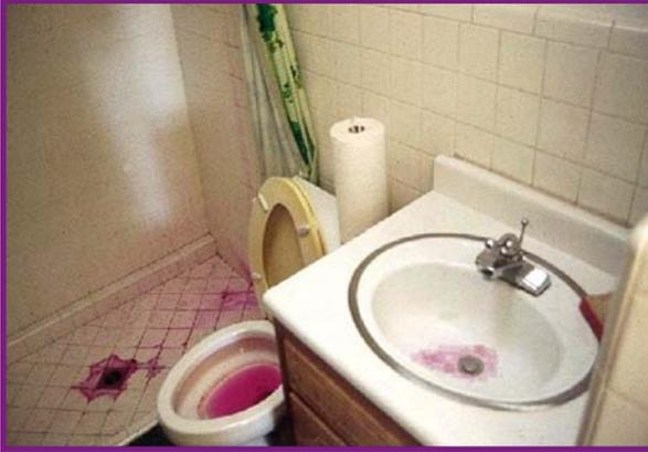
*Figure 5: Colored water in internal fixtures indicates a cross-connection*
