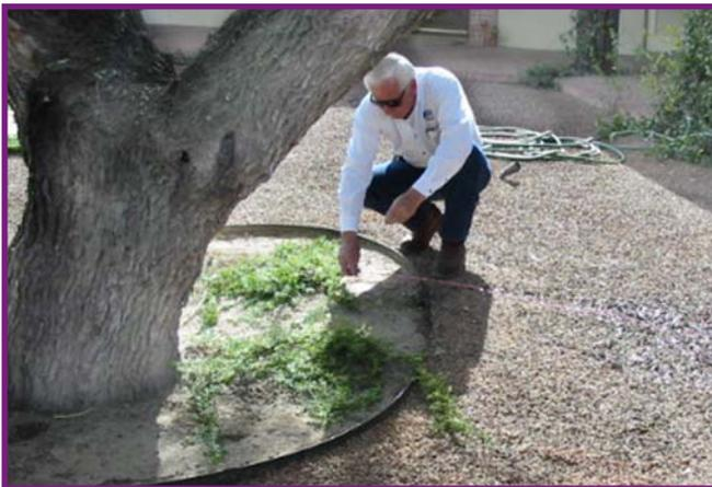
*Figure 4: All irrigation stations are checked for the presence of colored water*
