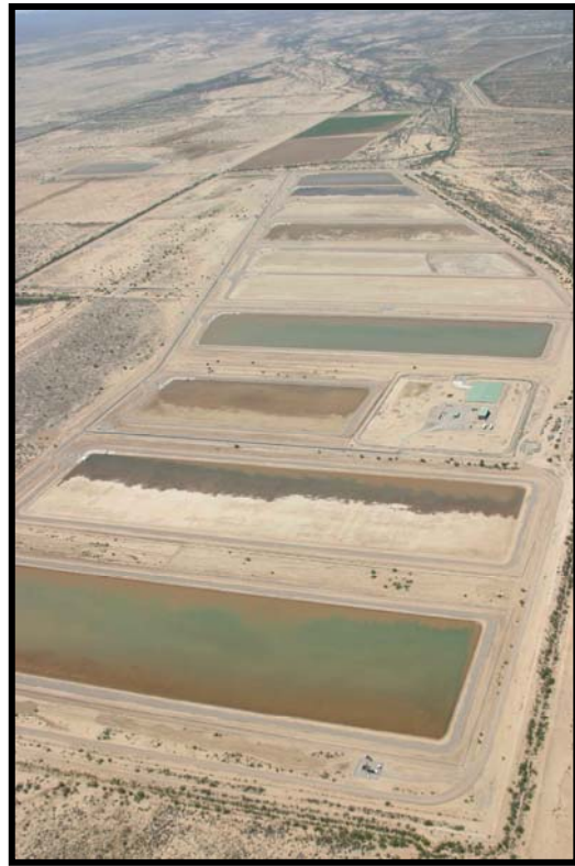
Basin Recharge of Colorado River Water – Tucson Water's Central Avra Valley Storage and Recovery Project went into operation in 2001.
